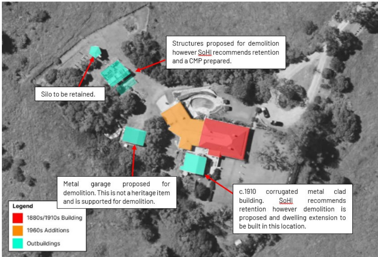
Figure 1: Structure identification image
