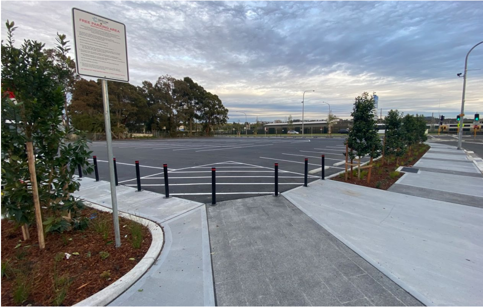
Dumaresq Street Car Park & Footpath, Campbelltown
