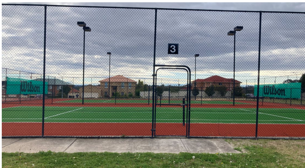
Tennis Court Surface Replacement
