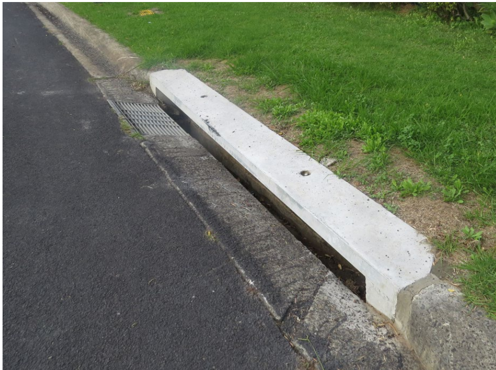
Stormwater pit lintel replacement at Tipping Place, Minto
