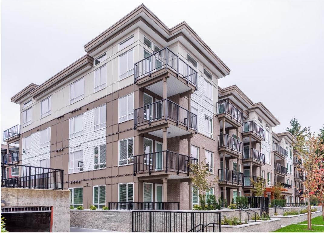
Figure 5.4 35 Dwellings / Hectare (R4 High Density) (illustrative purposes only – not to be taken as a control)
