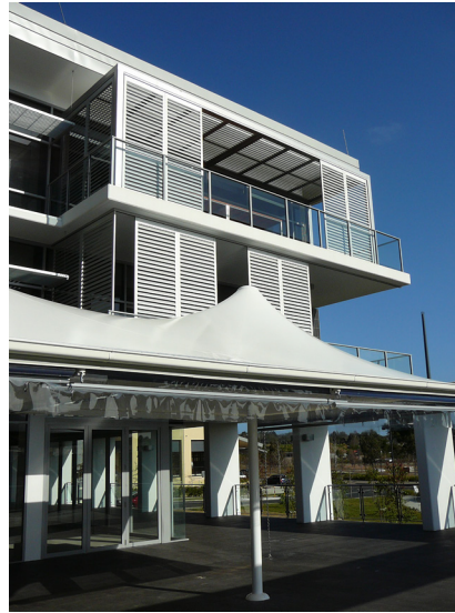
Figure 6.4.1.2 An example of a well articulated commercial building.
